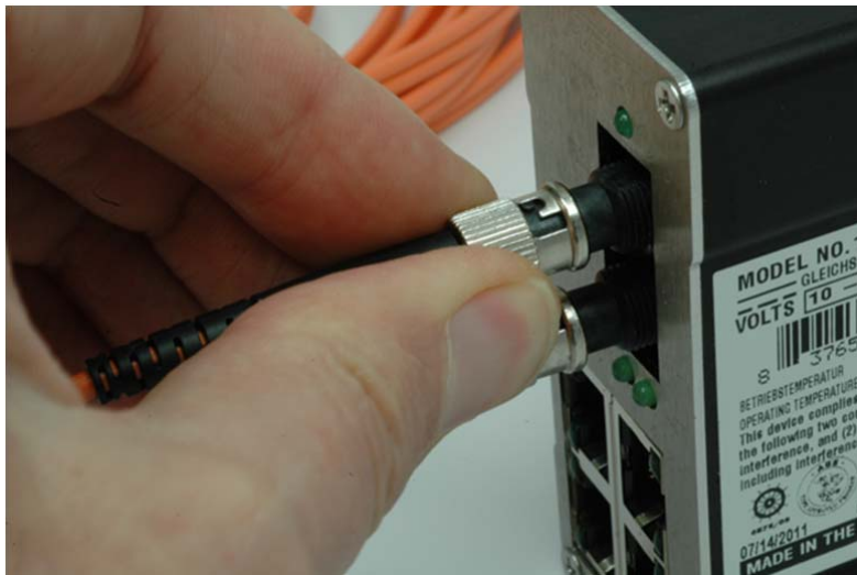
Figure 16: Connecting up the fibre
